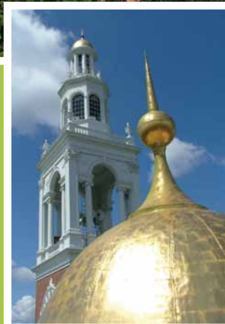
Dome and tower of Ira Allen Chapel at UVM following restoration.
