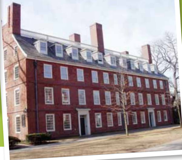
Massachusetts Hall, circa 1718, is the country's 2nd oldest continuously operating campus building. Dormitory to John Adams, John Hancock, and Sam Adams, it was designed for climate, with locally sourced brick, granite, and slate (key points – if only they had LEED certification back in 1718).
