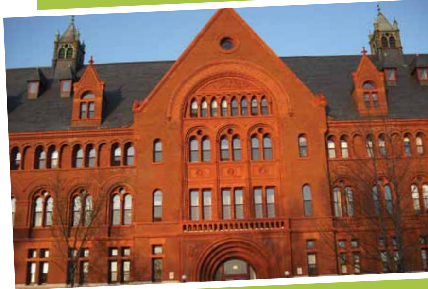
UVM's Williams Hall, circa 1896, is listed on the National Register of Historic Places following masonry, terra cotta, and window restoration to address building envelope and life safety issues.
