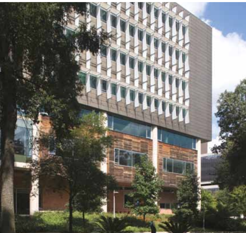
School of Nursing – looking southwest
