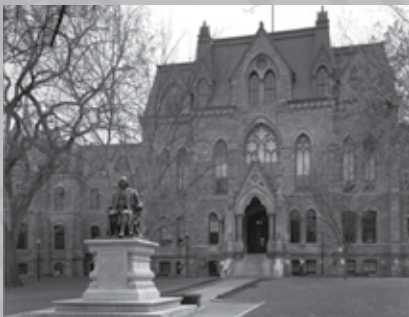
University of Pennsylvania Historic Stone Facade Repairs
