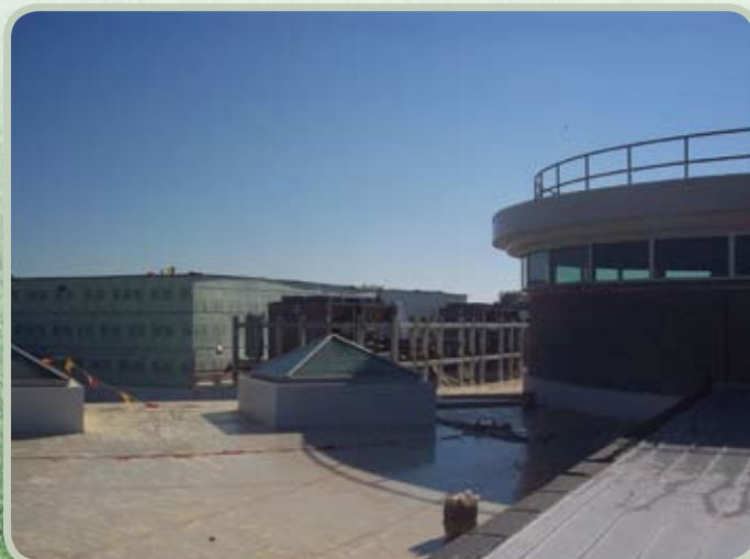
▲ Early construction of the facility rotunda, which is the central point of the Secondary Center.
