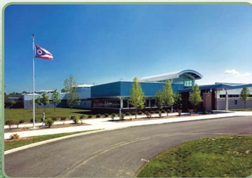
▲ The driveway into the Secondary Center at C-TEC.
