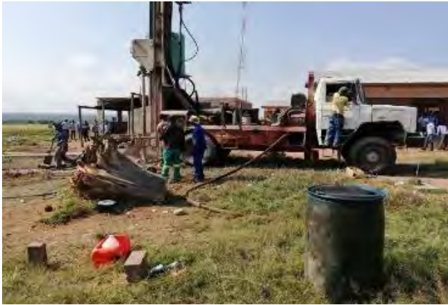
Figure 2. Upgrading the borehole to solve the water crisis
