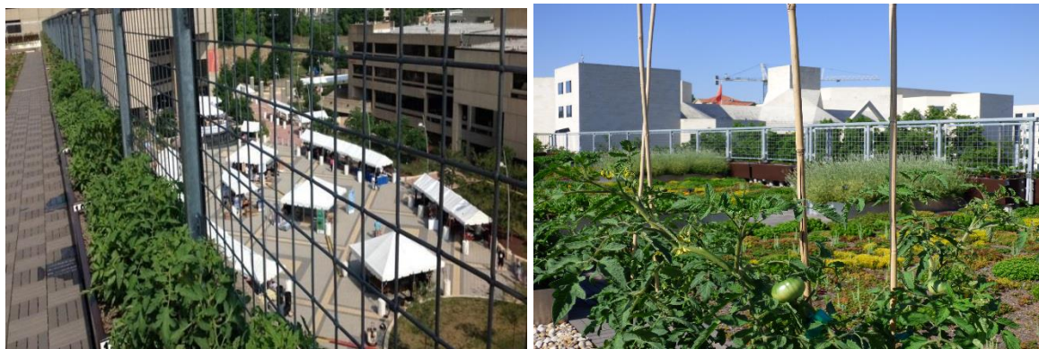
Figure 3. Food-Producing Green Roof of the UDC Van Ness Campus Urban Food Hub in Ward 3. Eighteen-inch deep planters placed around the perimeter of the roof support the production of a variety of food plants, from tomatoes to peppers, beans, okra, eggplant, and even berry bushes. The interior of the roof is limited to no more than four inches of soil depth, which can support the production of leaf lettuce, microgreens, and herbs. In its start-up phase the shallow beds are used mostly to grow sedums, a plant that is native to the area and requires little maintenance. The sedums absorb water and climatize the building, reducing storm water runoff and lowering heating and air conditioning needs (Horowitz, 2012; Whittinghill & Bradley Rowe, 2012).
