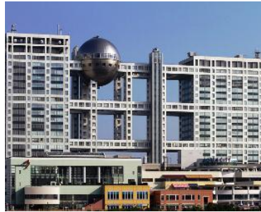
8. (H) Fuji TV building, Tokyo
