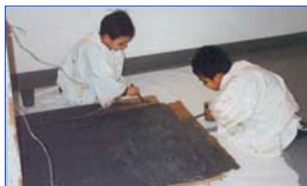
Figure 14. José and Felipe painted the lift.
