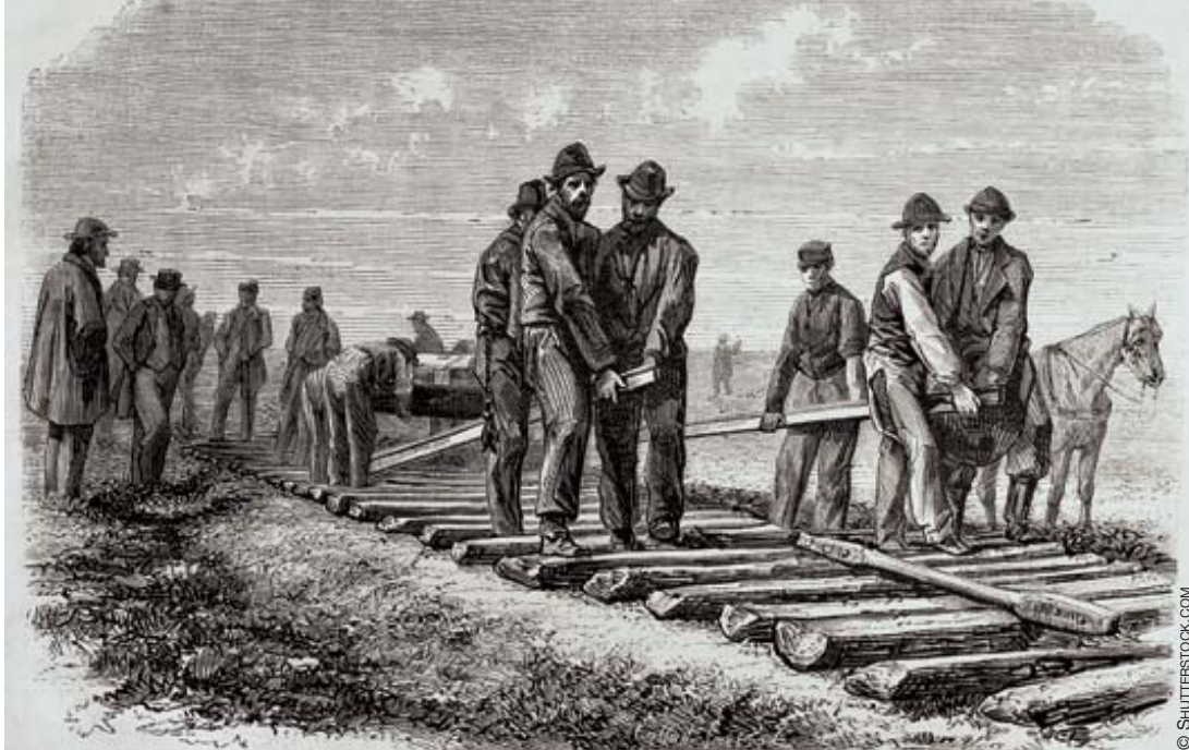
This antique illustration shows workers of the Union Pacific Railroad laying track for the transcontinental railroad that was completed in 1869.
