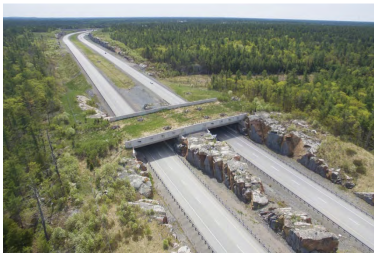
Figure 21. A Corridor Connecting Parts of the Habitat
