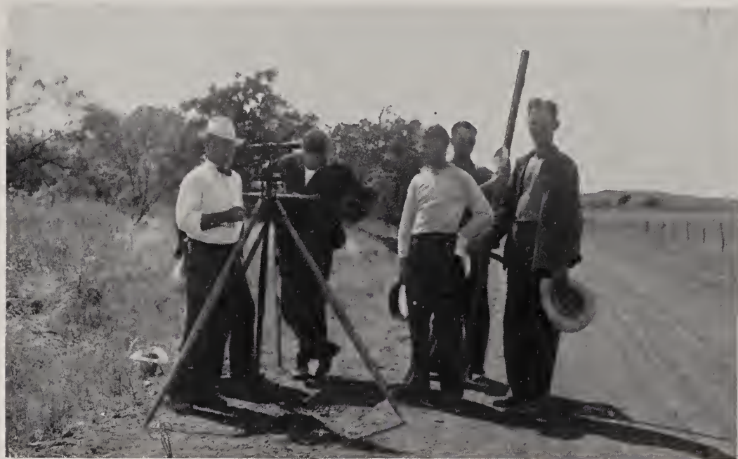
Enrollees learn surveying.
