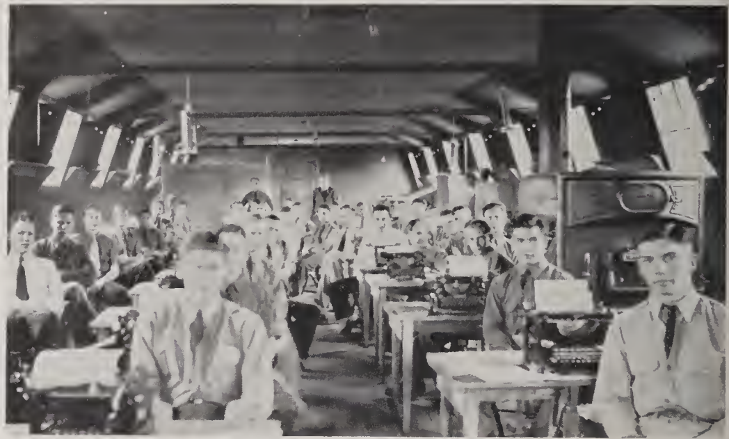
School for CCC company clerks.
