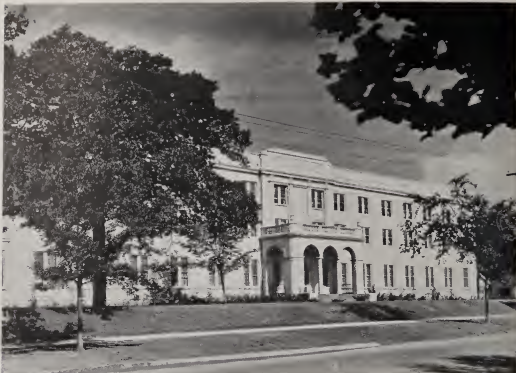
A new home for student teachers. $232,000 dormitory built on the campus of the Texas State Teachers College in Denton for 100 of its women students. It is one of a number of buildings constructed by the State College with allotments totaling $1,300,000 from the Public Works Administration.
