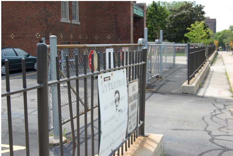
Picture 2. Securing the entry and access to the school facility.
