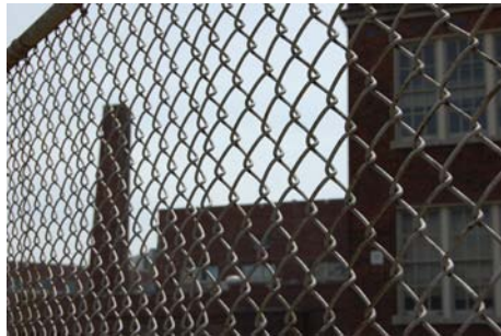
Figure 3. School Fencing (Elementary School)
