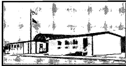
Two new 1,000 sq. ft. relocatable classrooms at Lawrence Township
