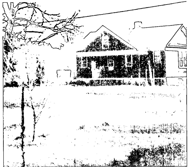
Raising the Roof: You may not need to if you are renovating an older school with a pitched roof. In 1991-1992 the spacious attic of the elementary school on Little Cranberry Isle, Maine, was turned into an apartment, which is currently rented to a teacher and his family on a 12-month basis. This is an important incentive for attracting teachers to this small coastal community in which there is a serious shortage of affordable housing, particularly in the summer. Photo courtesy of the Town of Cranberry Isle.
