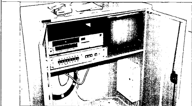
Monitoring equipment in secure cabinet
