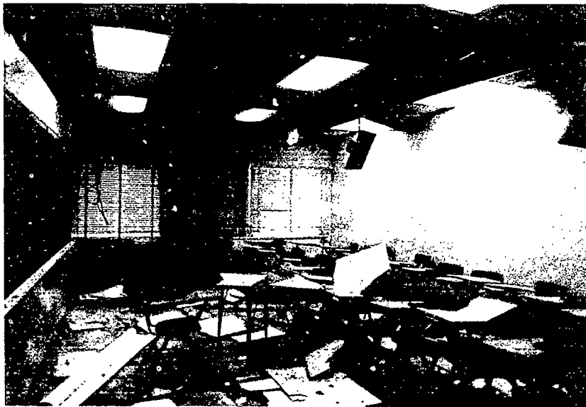
Fallen ceiling tiles in classroom at California State University, Los Angeles after the October, 1987 Whittier Narrows earthquake. (Photo provided by California State University, Los Angeles).
