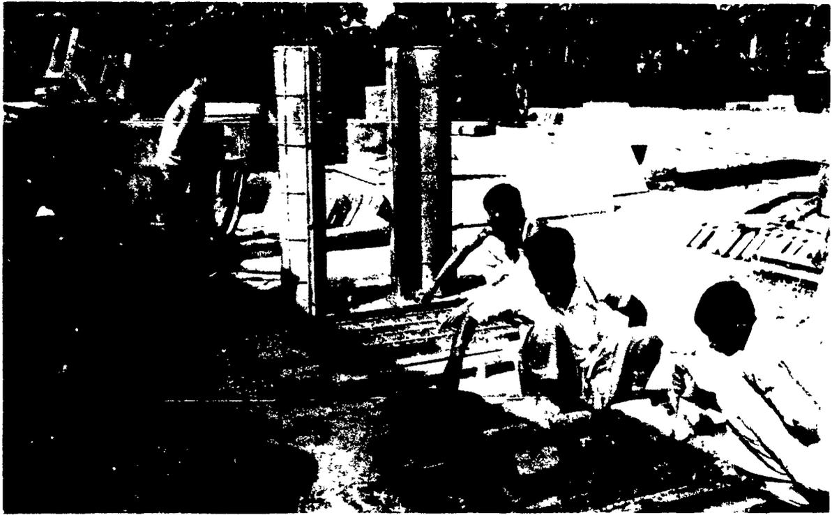
**Figure 17.** *Precasting of RCC elements: Columns are cast in the two vertical elements at the rear. In front of them a wall panel with bamboo reinforcement is being cast. In the foreground, a labourer is compacting the dry concrete mix around the forms which define the louvre openings.*
