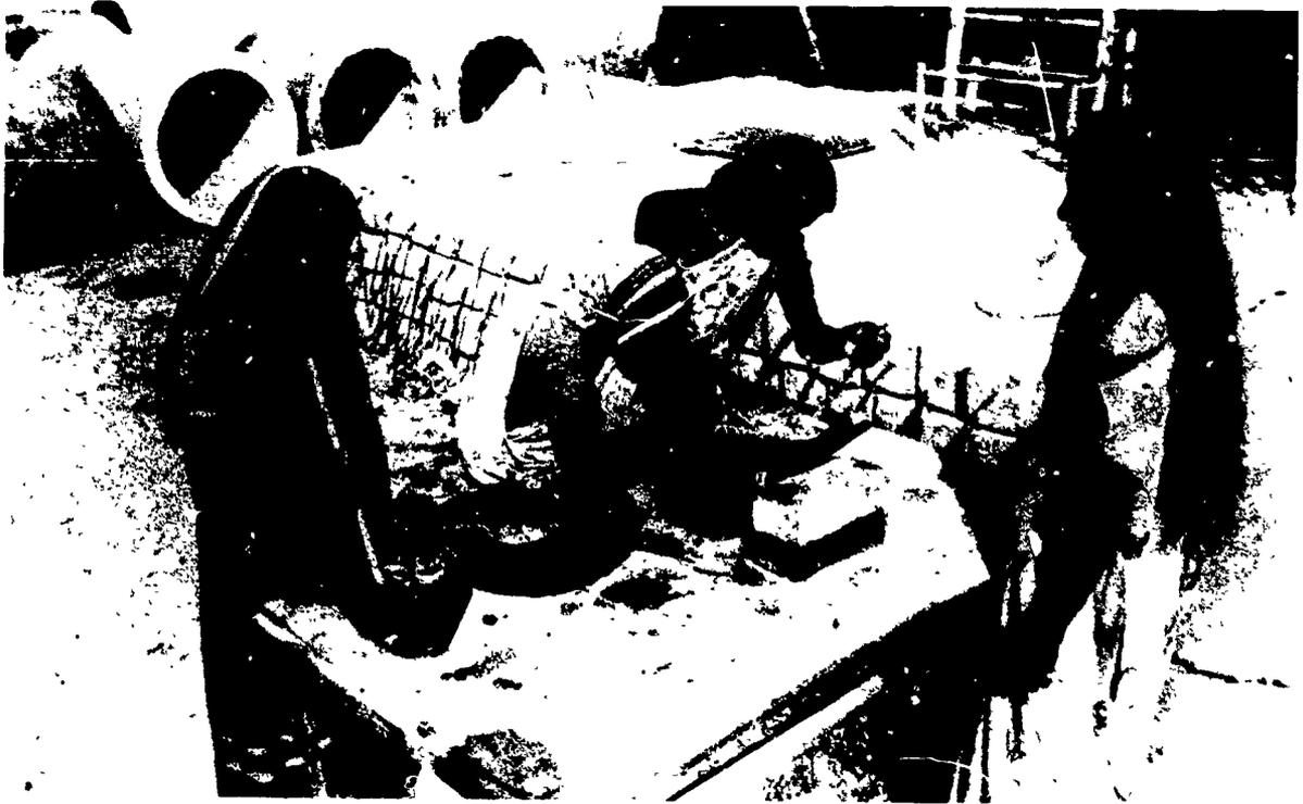
**Figure 19.** *Precasting toilet pan units. Two separate units are used to create a water seal toilet pan. Unskilled workers compact the concrete into the moulds.*
