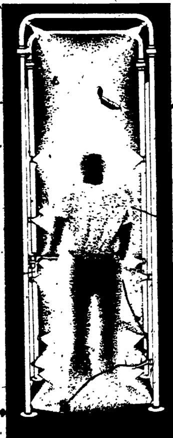
Figure 10. A safety shower is designed to wash a chemical off quickly, before it has time to act.
