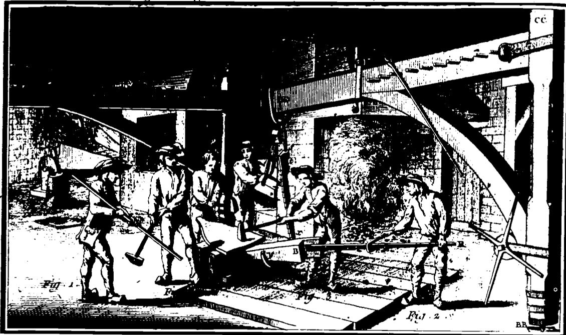
Blacksmiths forging an anchor.
