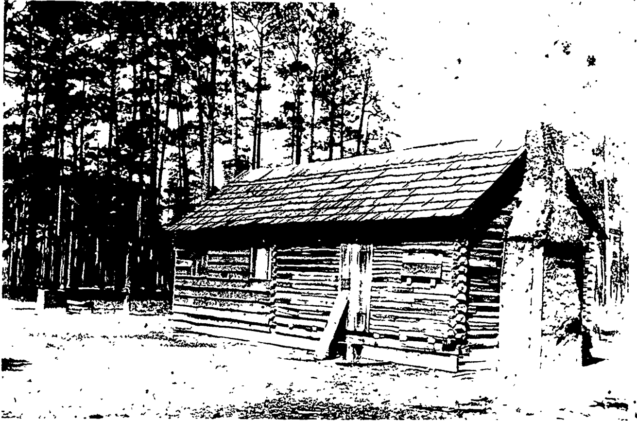
Eighteenth century log house with mud and wattle chimney, modern addition, and modern roof. Courtesy, Special Collections Department, University of Georgia Library.
