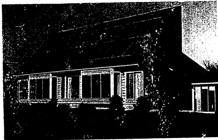
**Figure 14** *This experimental four-bedroom, full-basement house at the University of Delaware obtains 80% of its power, heat, and air conditioning from the sunshine that falls on its roof and front walls. Part of this is converted directly to electricity, with a reserve stored in batteries; part is stored as heat in a 6-foot cube of special salts from which heat is withdrawn as needed.*
