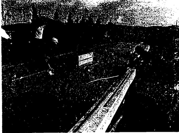
**Figure 20** *At ERDA's Lawrence Livermore Laboratory in California, water passing slowly through these shallow ponds, which are insulated and covered with plastic, is heated by the sun up to 170°F. This hot water is estimated to cost one-third as much as fuel-heated water. The possibilities of its practical use for industrial processes, or to boil a refrigerant fluid to turn a turbine and generate electricity, are being investigated.*
