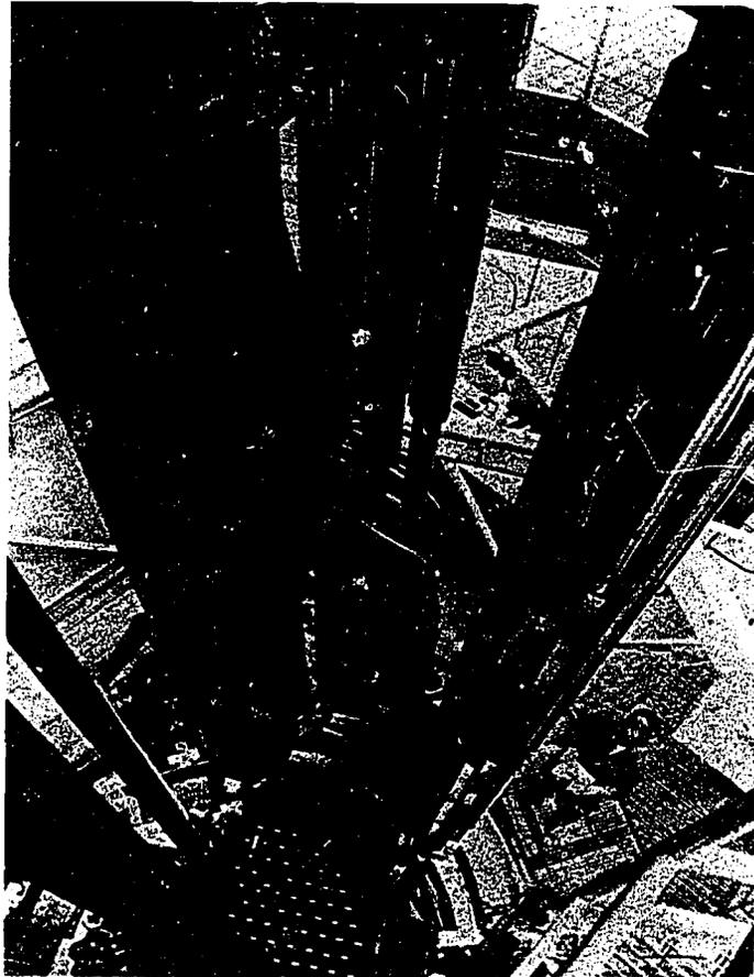
*This array of instruments will monitor the behavior of nuclear fuel during reactor operations. It is one component of the Fast Flux Test Facility now being constructed at Hanford, Washington. This original and innovative research and development facility will provide experience in designing, fabricating, and operating liquid metal fast breeder reactors, which would hold down the cost and extend the supply of uranium fuel.*
