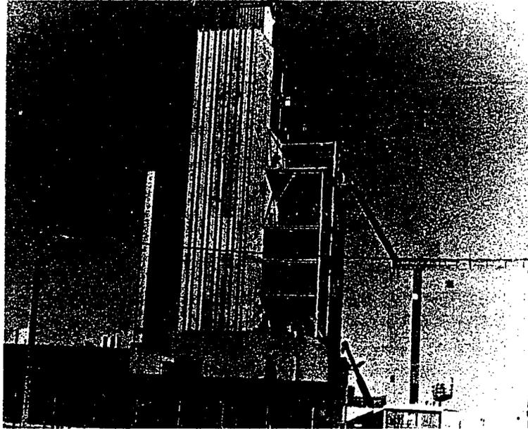
*An ERDA plant at Rapid City, South Dakota, is testing a process to convert lignite and other more reactive coals to high BTU gas. This concept, called the CO<sub>2</sub> Acceptor Process, involves the reaction of crushed limestone with carbon dioxide, one of the byproducts of gasification. The reaction, which releases the heat needed to keep the gasification process going, results in a synthetic gas enriched in methane and hydrogen.*
