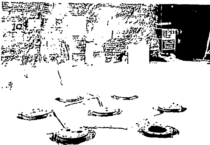
Photo C. Holes, 12 feet deep and lined with stainless steel, in the salt mine floor are used to contain radioactive fuel assemblies. The room is 30 feet wide, 60 feet long, and 14 feet high.
