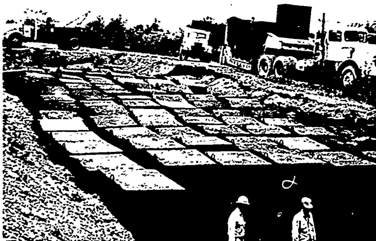
Figure 11 Land burial trench at the Oak Ridge National Laboratory reservation. Each day's accumulation of waste containers is buried by 3 or more feet of earth.
