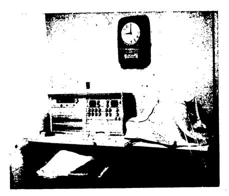
An inter-communication system links the entire school together. Also records, tape recordings and radio can be channelled to one or any number of spaces in the building. Conduit is in so future closed circuit instructional television is possible.
