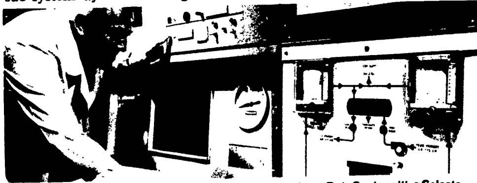
The ultimate in modern control: a Honeywell Supervisory DataCenter with a Selectographic console to monitor all of your important building operational systems
