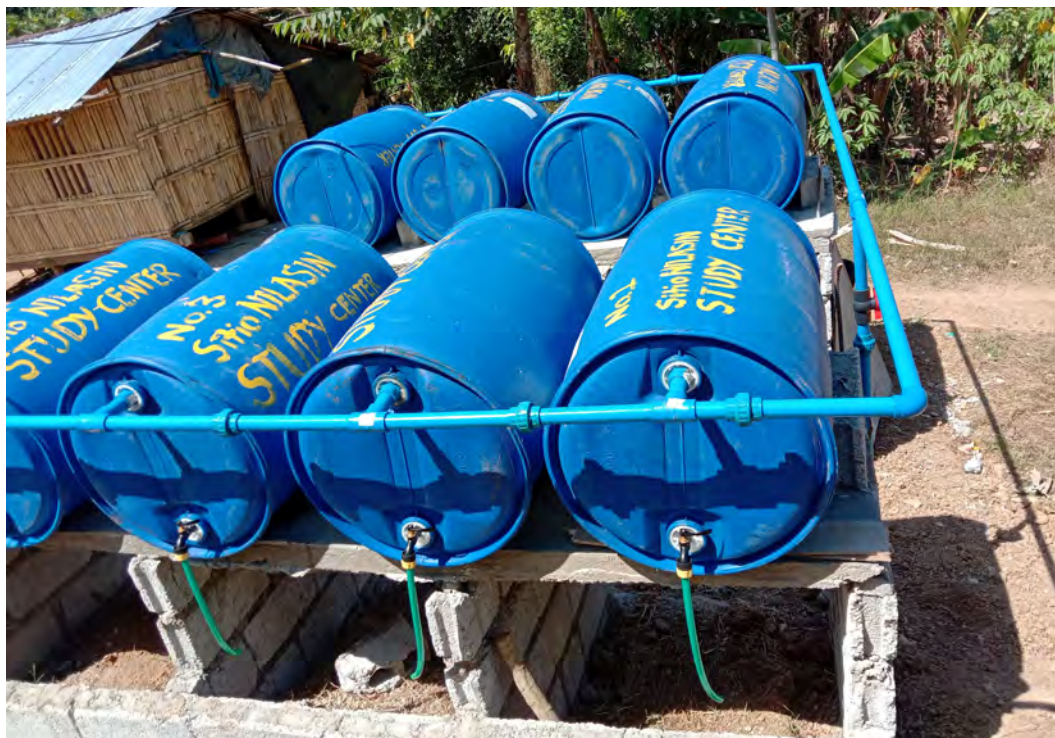
Figure 2. Water System Installed to Provide Water to Aeta Families
