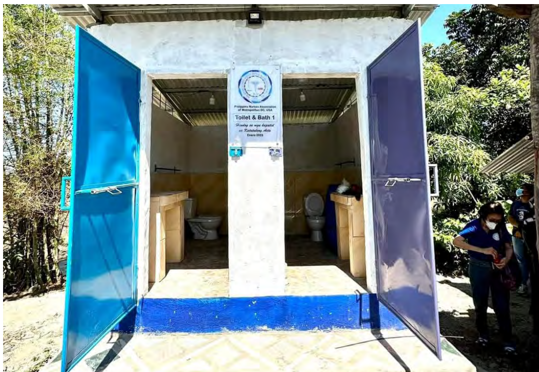
Figure 6. Baths Constructed for the Aeta Families in Mambagan
