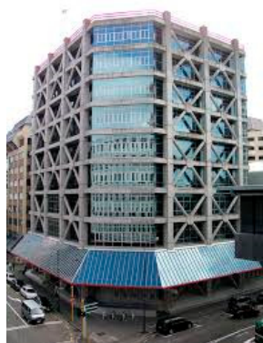
Figure 2. Bracing on building in Christchurch, NZ after an earthquake.
