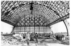
Figure 6: Nervi's Aircraft hangar (BMIAA,2017)
