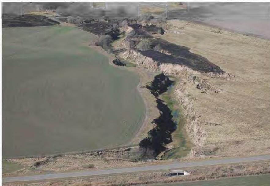
Figure 6. Regressive erosion gully in Arroyos Menores area
