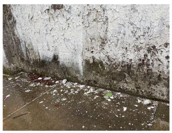
*Figure 3*. Sidewalks are littered with paint chips from dilapidated viaducts
