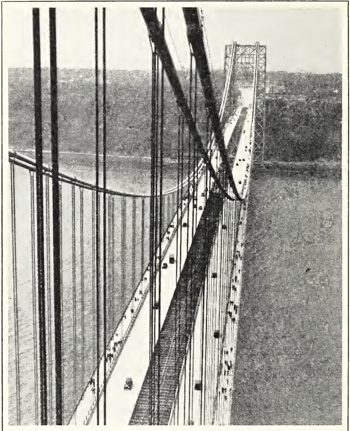
FIG. 154. Engineers in Building a Bridge must allow for the Expansion and Contraction of Cables Such as These
