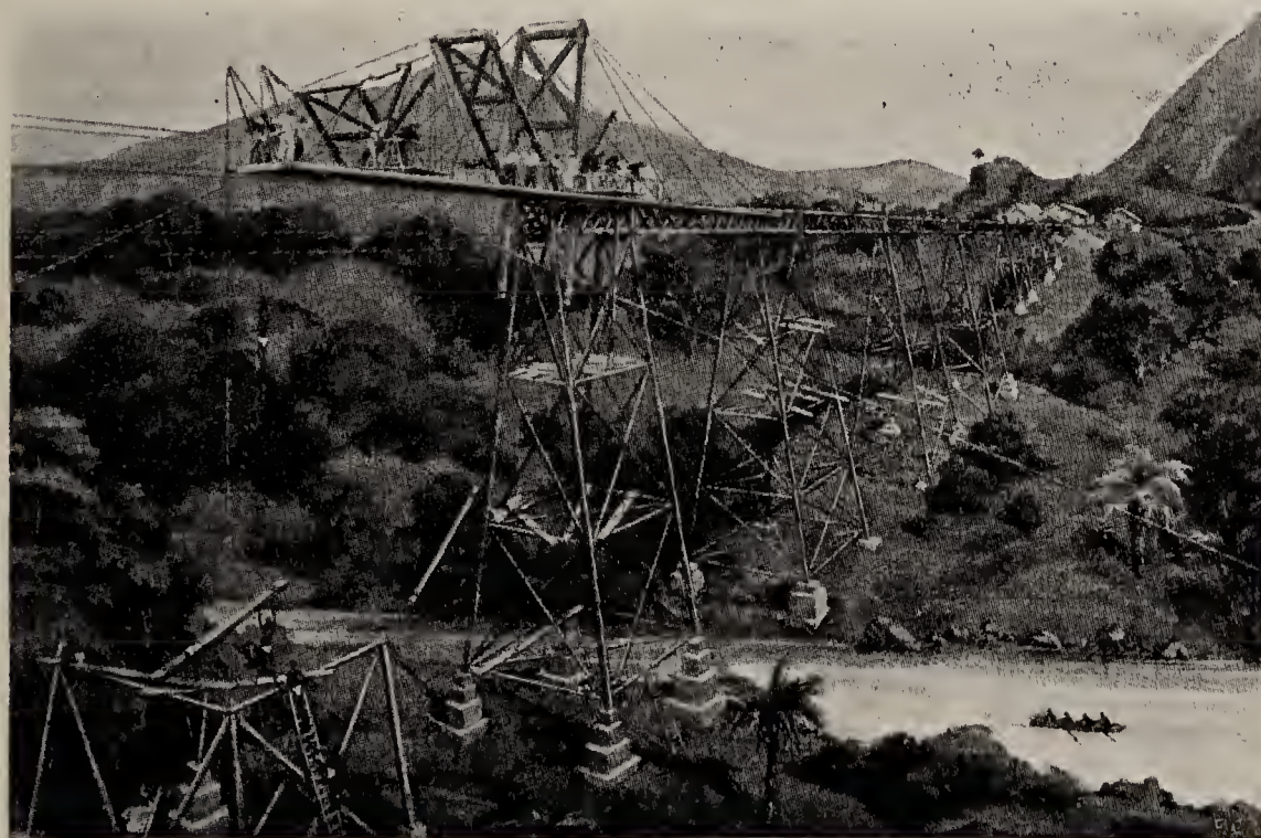
CONSTRUCTION OF RAILWAY BRIDGE IN SIERRA LEONE, WEST AFRICA
