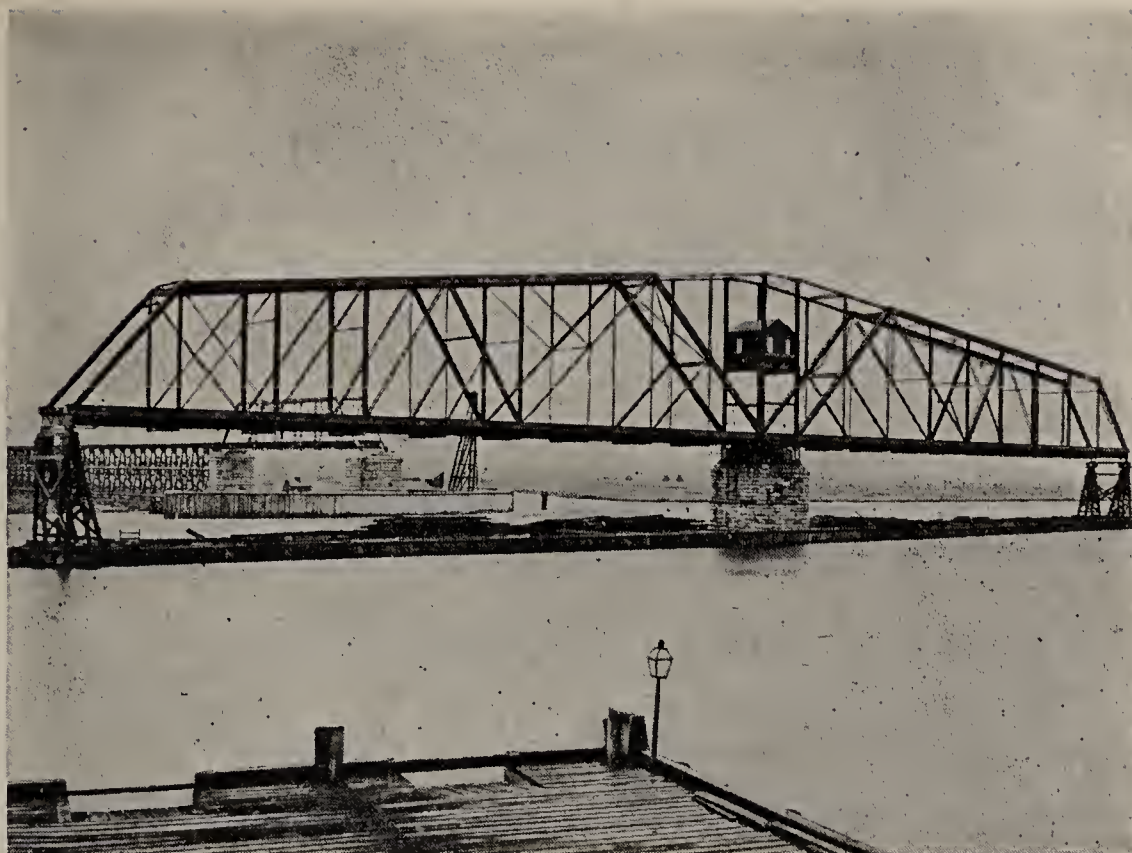
PHOTOGRAPH OF 500-DRAW SPAN, SHOWING CHANNEL OPEN
