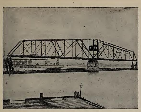
PHOTOGRAPH OF 500-DRAW SPAN, SHOWING CHANNEL OPEN
