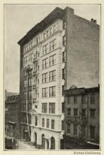
Sandblasting. Note the difference between the part of the building that has been sandblasted and the part that has not yet been cleaned.
