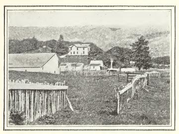
This fence was built in a straight line. You can see what happened to it during an earthquake<sup>1</sup>
