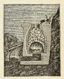
FIG. 90.—Lime-kiln. When calcarecus stones are subjected to a very high temperature they are transformed into lime.
