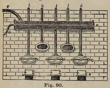
placed in a single furnace. Each one, after receiving a charge of from one hundred pounds to one hundred and fifty pounds, is closed airtight as shown at G, and made red-hot by the fire in the furnace, whose doors are shown at A. In
