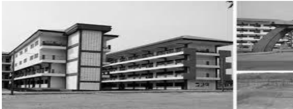
Figure 2. An E-Block senior high school building in Ghana
