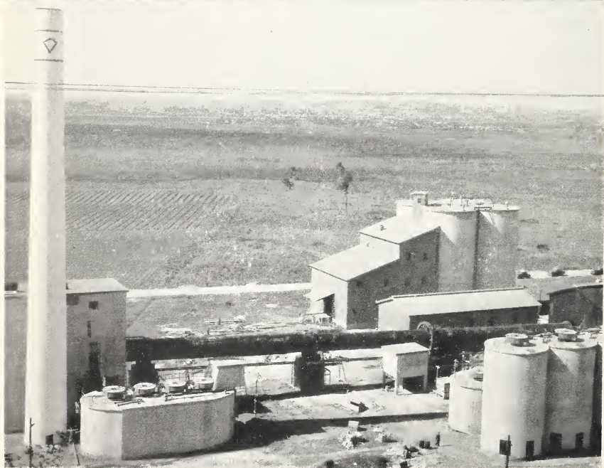
UPPER: A SEMIURBAN LOW-COST HOUSING DEVELOPMENT IN PUERTO RICO. LOWER: A CEMENT PLANT CONSTRUCTED BY THE PUERTO RICO RECONSTRUCTION ADMINISTRATION.
