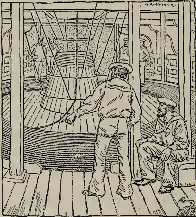
PAYING OUT THE CABLE FROM THE HOLD OF THE GREAT EASTERN
