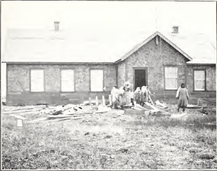
GOVERNMENT SCHOOL BUILDING AND TEACHER'S RESIDENCE. WAINWRIGHT.
