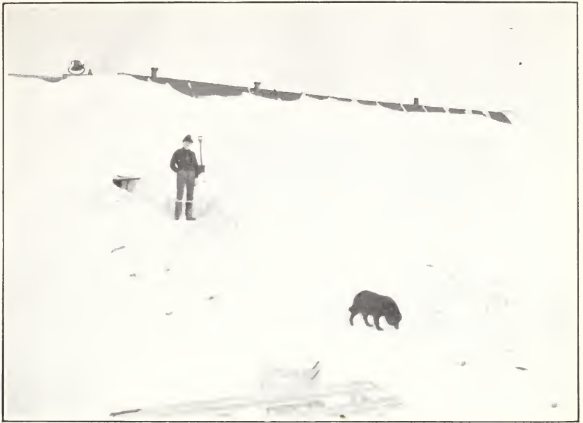
Tunnel to door.
