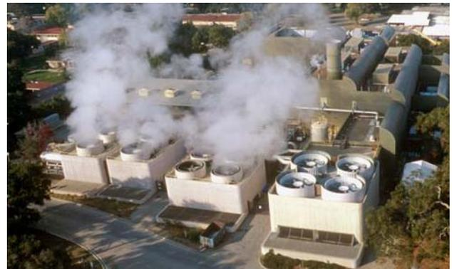
*Stanford's on-site cogeneration facility provides electricity, steam, and chilled water to campus buildings. Operating as its own utility, Stanford is also able to offer rebate programs comparable to local public utility companies, a factor which helped to support the creation of the ERP and the WBERP.*
