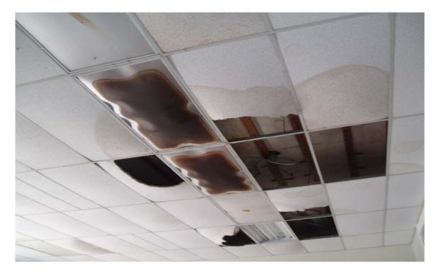
Water damage to ceiling
