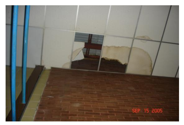
Wet, damaged ceiling tile
