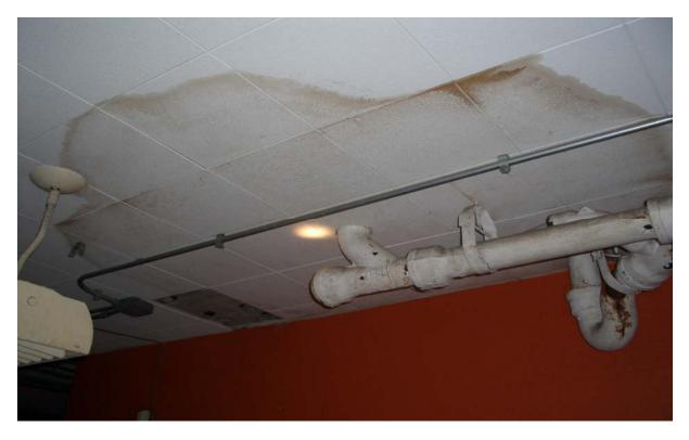
Water damage in ceiling tile
