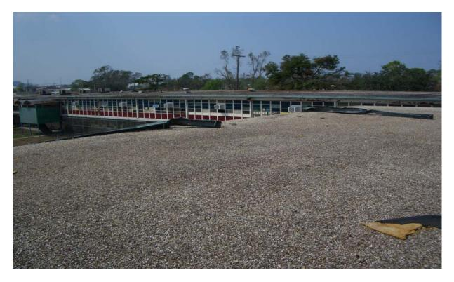
Gutters blown up onto roof
