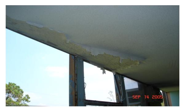
Ceiling damaged by wind & water
