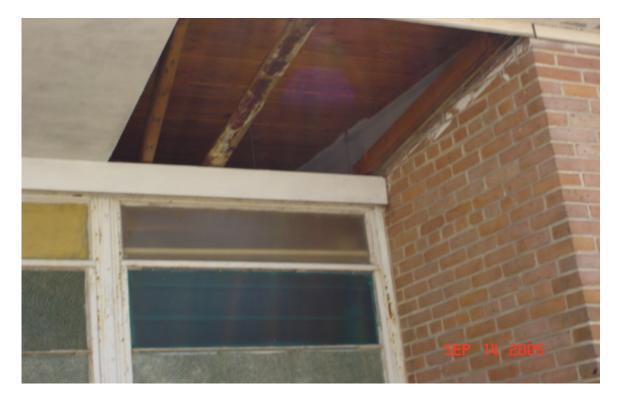
Soffit missing, front
