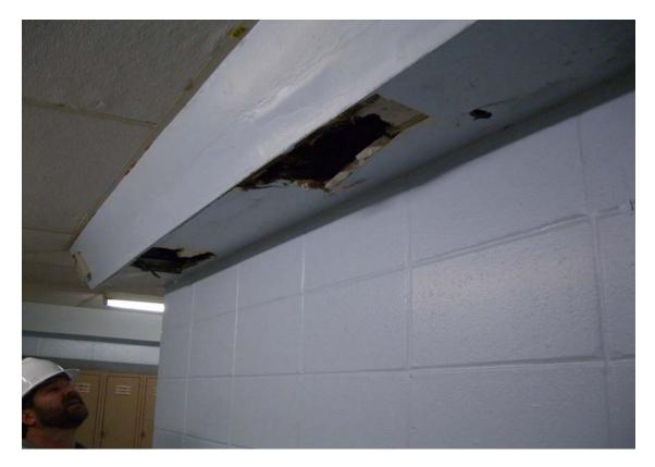
Water damage in duct, evidence of mold
