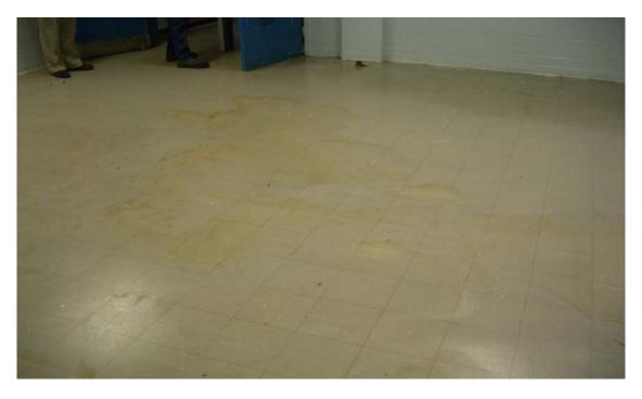
Water damage on floor by entranceway
