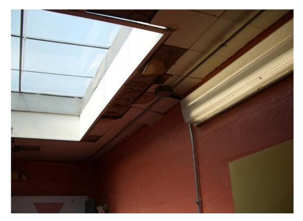
Ceiling tile water damage in stairwell
