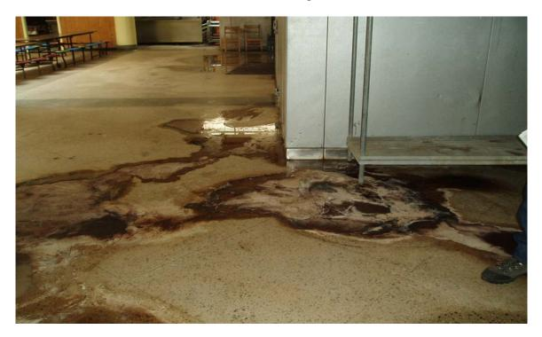
Water damage to floor
