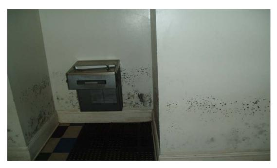
Water damage and mold
