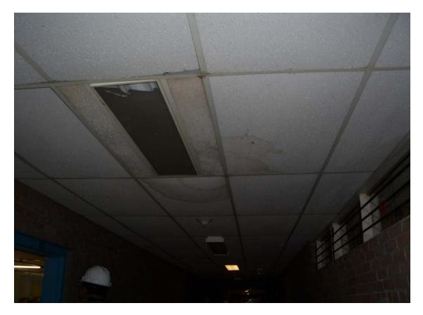
Water damage to ceiling in hallway
