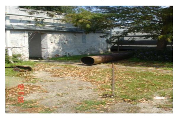
Boiler stack blown off boiler building
