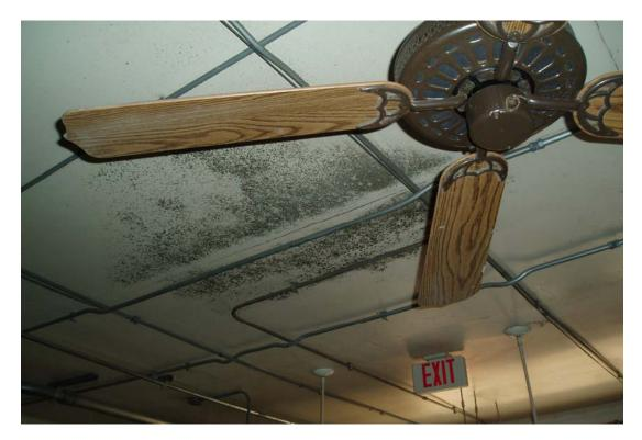
Evidence of water damage and mold
