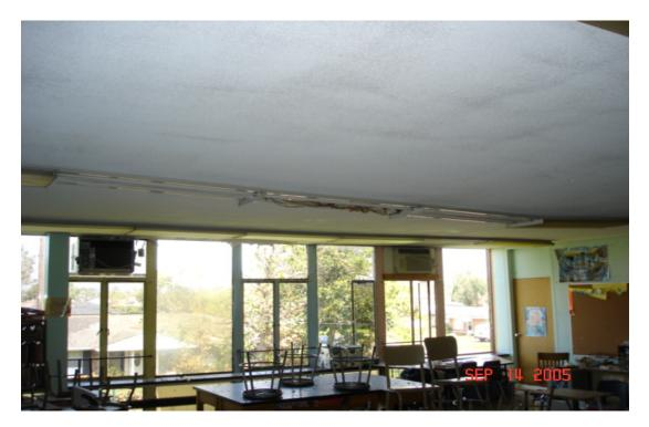
Damaged Ceiling – Room not safe to occupy
