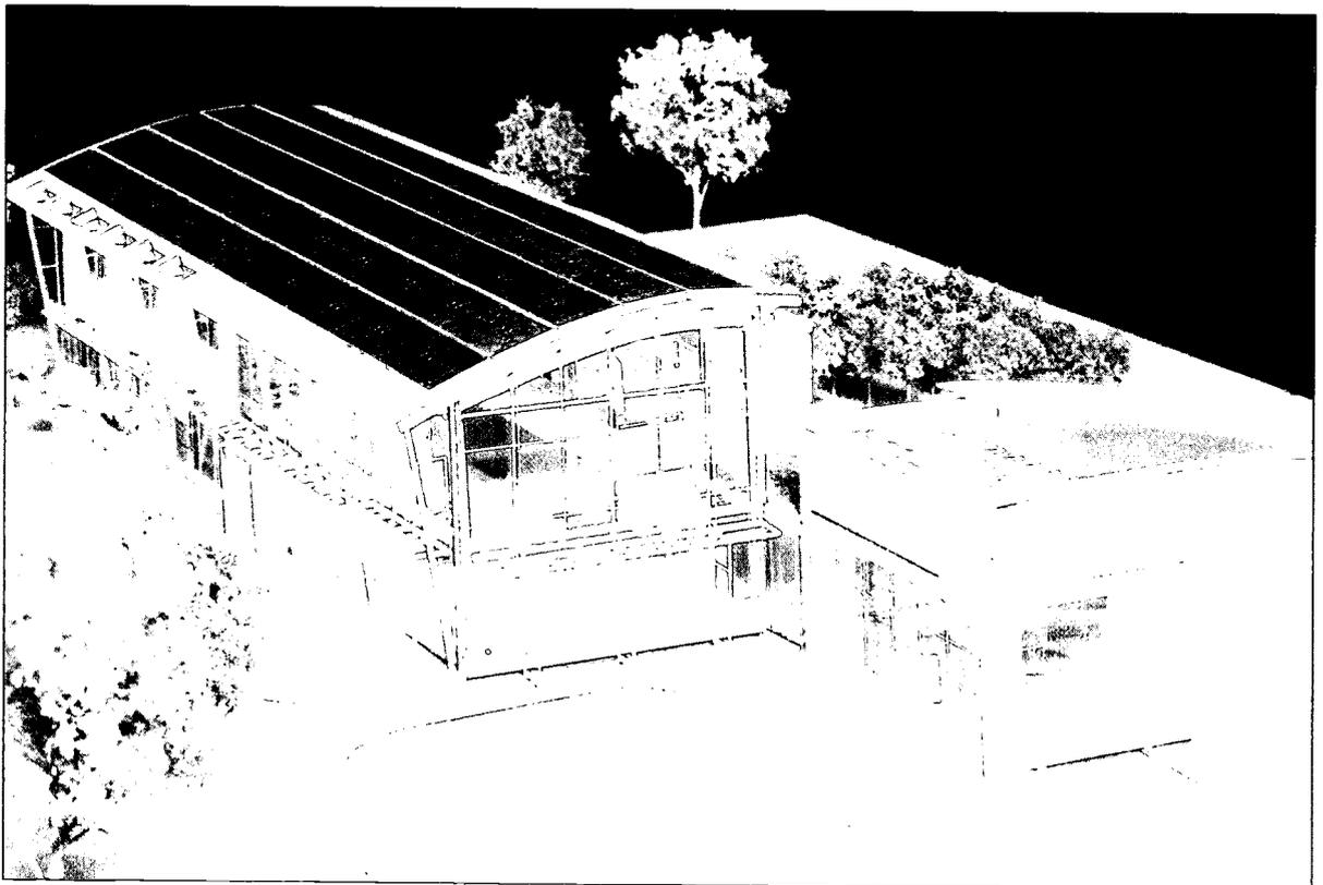
*Architect's model of the Lewis Center at Oberlin College. PV panels cover the dark area of the main roof.*
