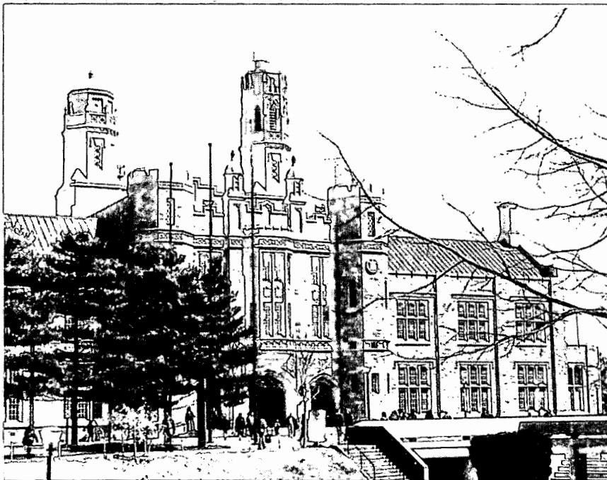
Music Building at Lehman College
