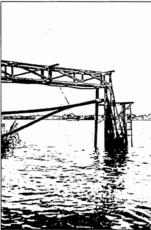
This water pipe is used to pump water from the Volta River to the town of Adidome, where people then fetch water from the standpipes. The Volta River is downstream from the dam that created the largest manmade lake in the world. Damming the river has damaged its ecology; however, the dam is used for creating electricity in the area.
