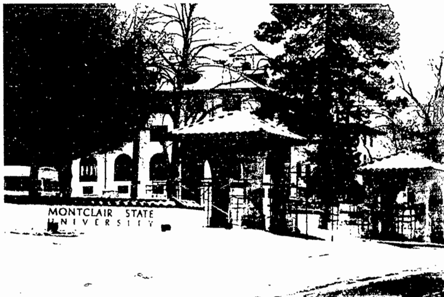
Construction at the Normal Avenue Entrance, Montclair State University
