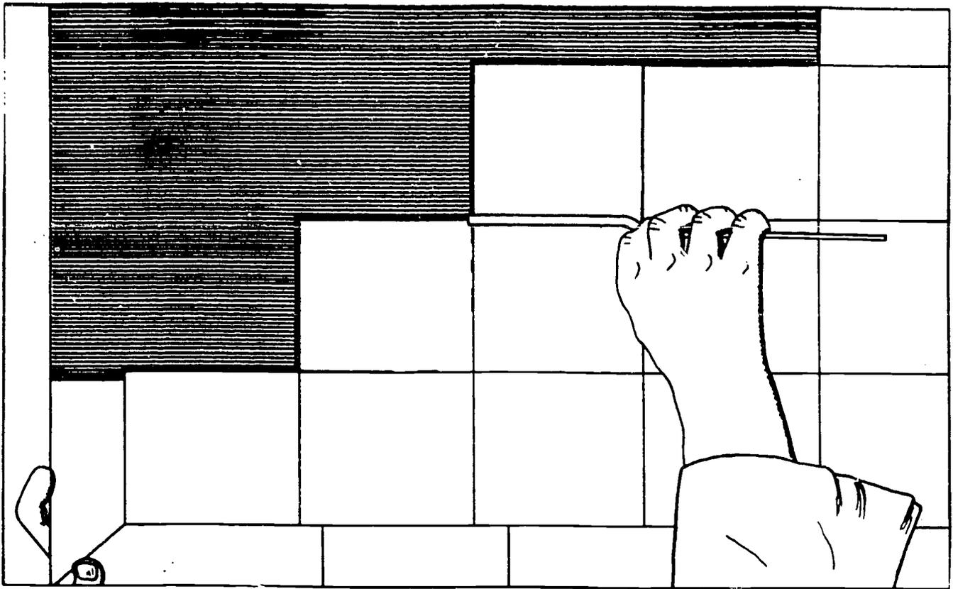
Figure 56. Jointing Grouted Tile Joints
