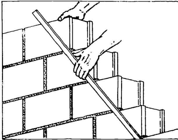
Figure 6. Checking the Horizontal Spacing
