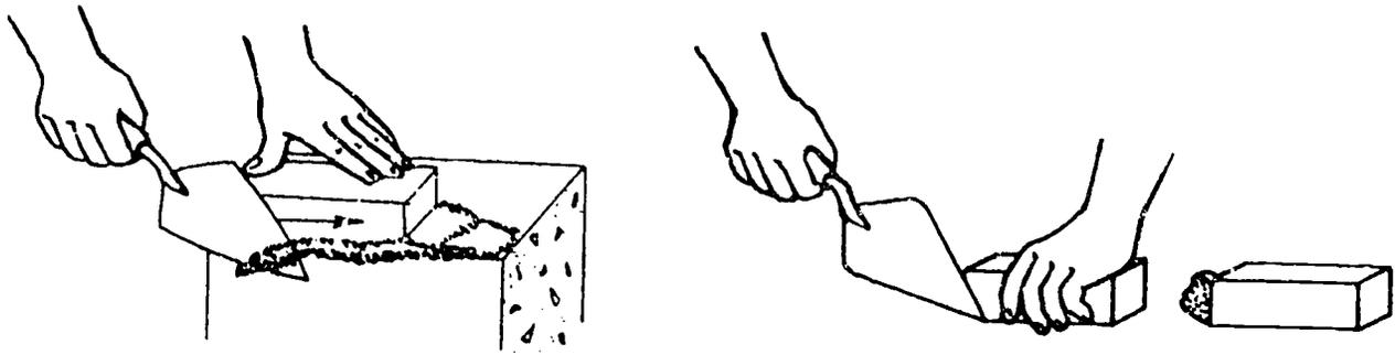
Figure 22. Cutting Off Mortar and Buttering a Stretcher
