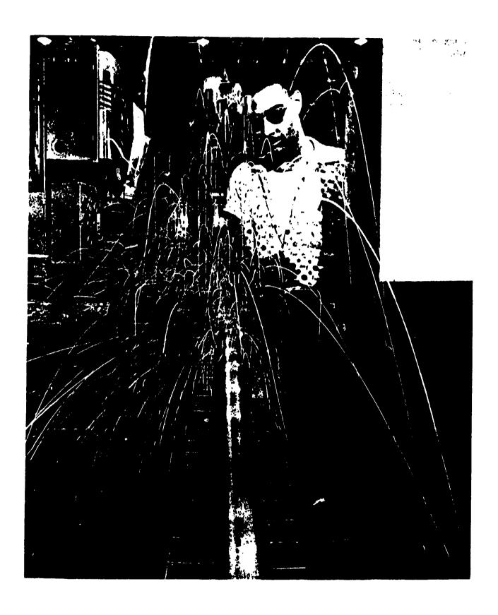
Welding Studs to Tubes (The Babcock and Wilcox Co.)
