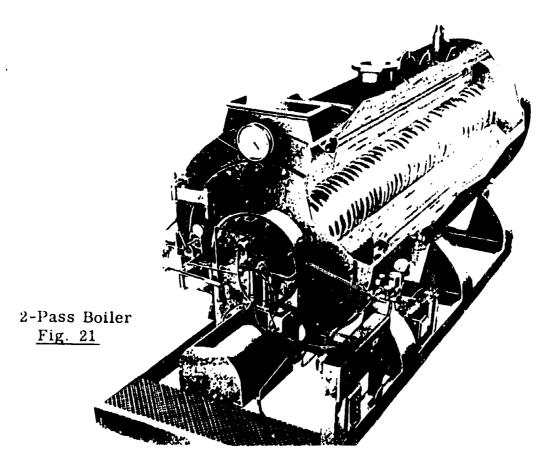
This 2-pass design features a corrugated furnace of generous proportions to minimize radiant transfer from a highly turbulent flame. The second pass consists of two staggered rows of relatively widely spaced return tubes.
