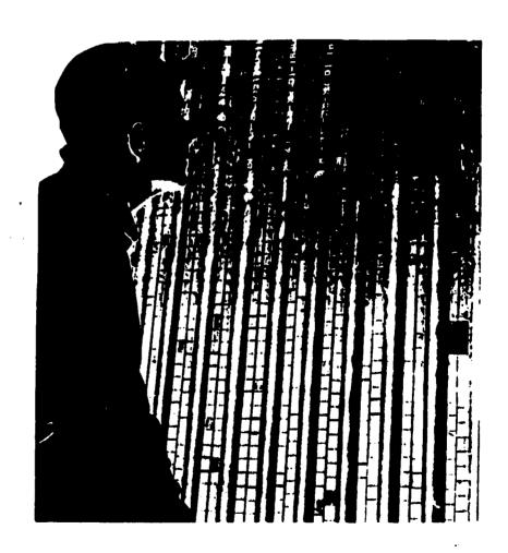
Flat-Stud Tube Wall (Furnace Side) (The Babcock and Wilcox Co.)
